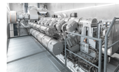
The 35/44G TS can be operated with synthetic climate-neutral fuels
