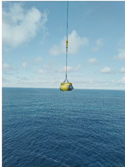
Radial barrel compressor bundle during loading on Equinor's Troll A platform, Norwegian North Sea © Everllence
