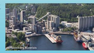
Around 440,000 tons of CO<sub>2</sub> annually and approx. 50 percent of the Brevik plant's total emissions are captured, compressed, liquefied and transported by ship to Bergen (western Norway). From there, a pipeline leads to an underground storage location in the North Sea. Taking into account the life-cycle greenhouse gas emissions of the entire process chain (capture, compression and transport), this results in a net emission reduction of around 330,000 tons of CO<sub>2</sub> per year.
